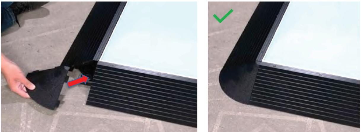
10. Slot the corner ramps in place at each corner of the panel assembly. It can be helpful to lift both adjacent edge ramps slightly in order to align the corner ramp, the edge ramps, and the connection bracket. Once aligned, the three ramp pieces should fall easily into place.
